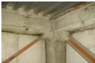
吹付け材の例(梁・柱)
